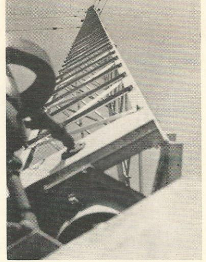
ABOVE: Looking up the 185-foot radiator installed at "Vagabond" in Seoul, across the base insulator and the Austin tower lighting transformer.
