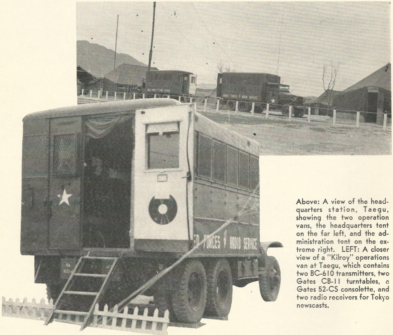
Above: A view of the headquarters station, Taegu, showing the two operation vans, the headquarters tent on the far left, and the administration tent on the extreme right. LEFT: A closer view of a "Kilroy" operations van at Taegu, which contains two BC-610 transmitters, two Gates CB-11 turntables, a Gates 52-CS console, and two radio receivers for Tokyo newscasts.
